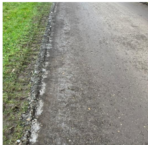
Stabilised Roadway ready for Surfacing
