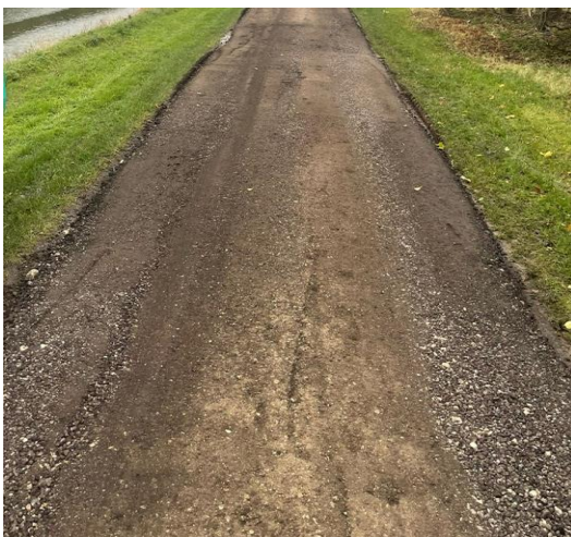
Roadway Trimmed level and ready for Stabilisation
