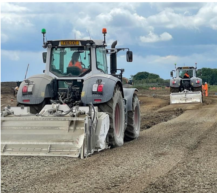
7A Soil being mixed after mellowing with Lime
