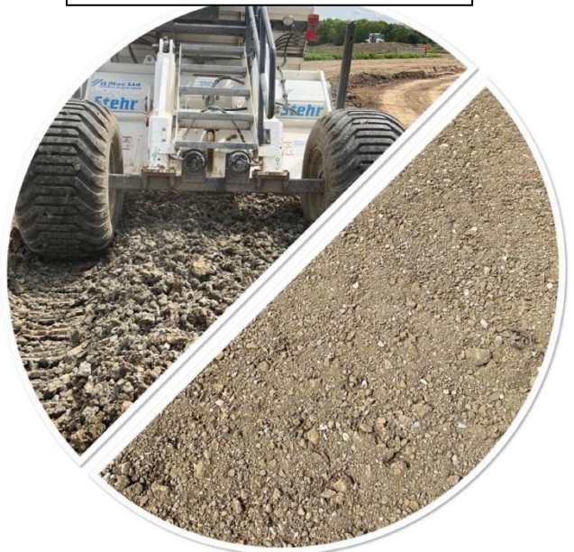
7A material ready for Cement Stabilisation
