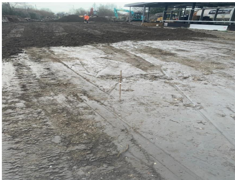
Stockpile material Placed and Cement Mixed in Layers
