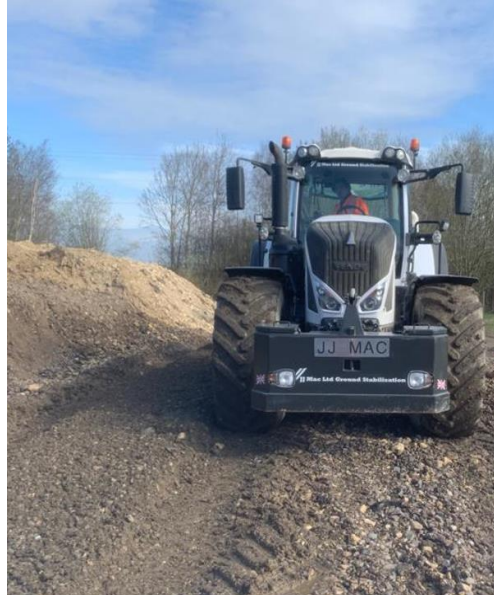
Ex-Situ Cement Mixing
