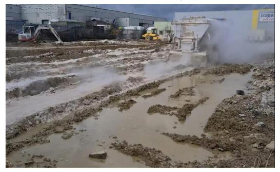
• The works had a two-fold advantage to this site. **JJMac Ground Stabilisation Dried** the site out, saving programme time. The 300mm cement layer (once capped with Type1) served as a **Piling and Working Platform** to allow the site works to continue in dry clean conditions
